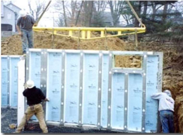
Window rough opening.
