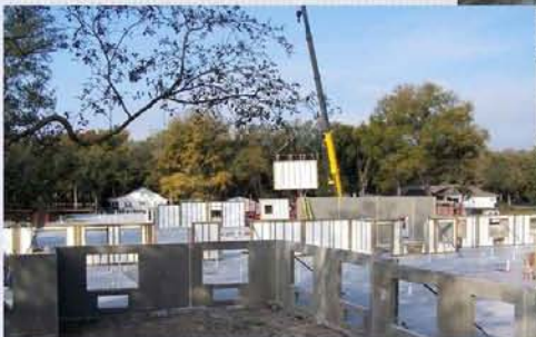
Epic Wall Panel Installing
