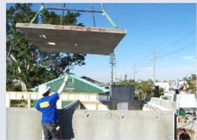
Safe Room Ceiling
