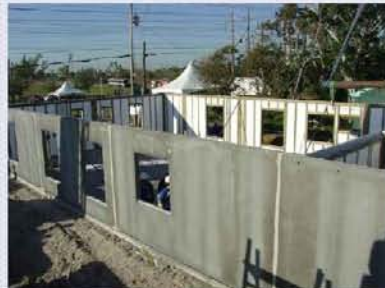
Epic Walls Installed in 2.5 hours
